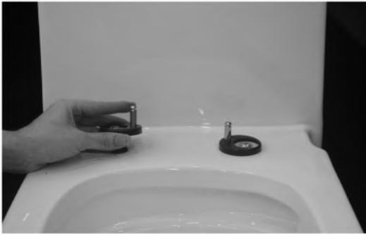
1. Insert the screws on the hinge base and then into the holes on the pan.
