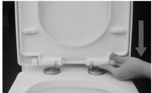
4. Try the seat on the hinges, re-adjust it if the distance does not match until it fits. Take off the metal cover and tighten the screws
