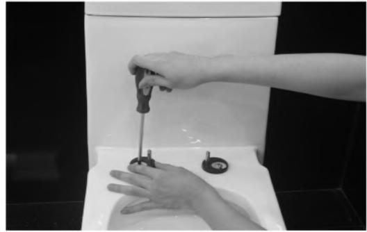
2. Tighten the screws to fix the hinge bases (but not fully tightened at this stage)
