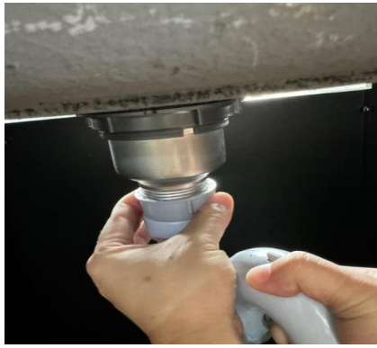
Rotate the drainer to secure it in the bottom of the outlet funnel(1)
